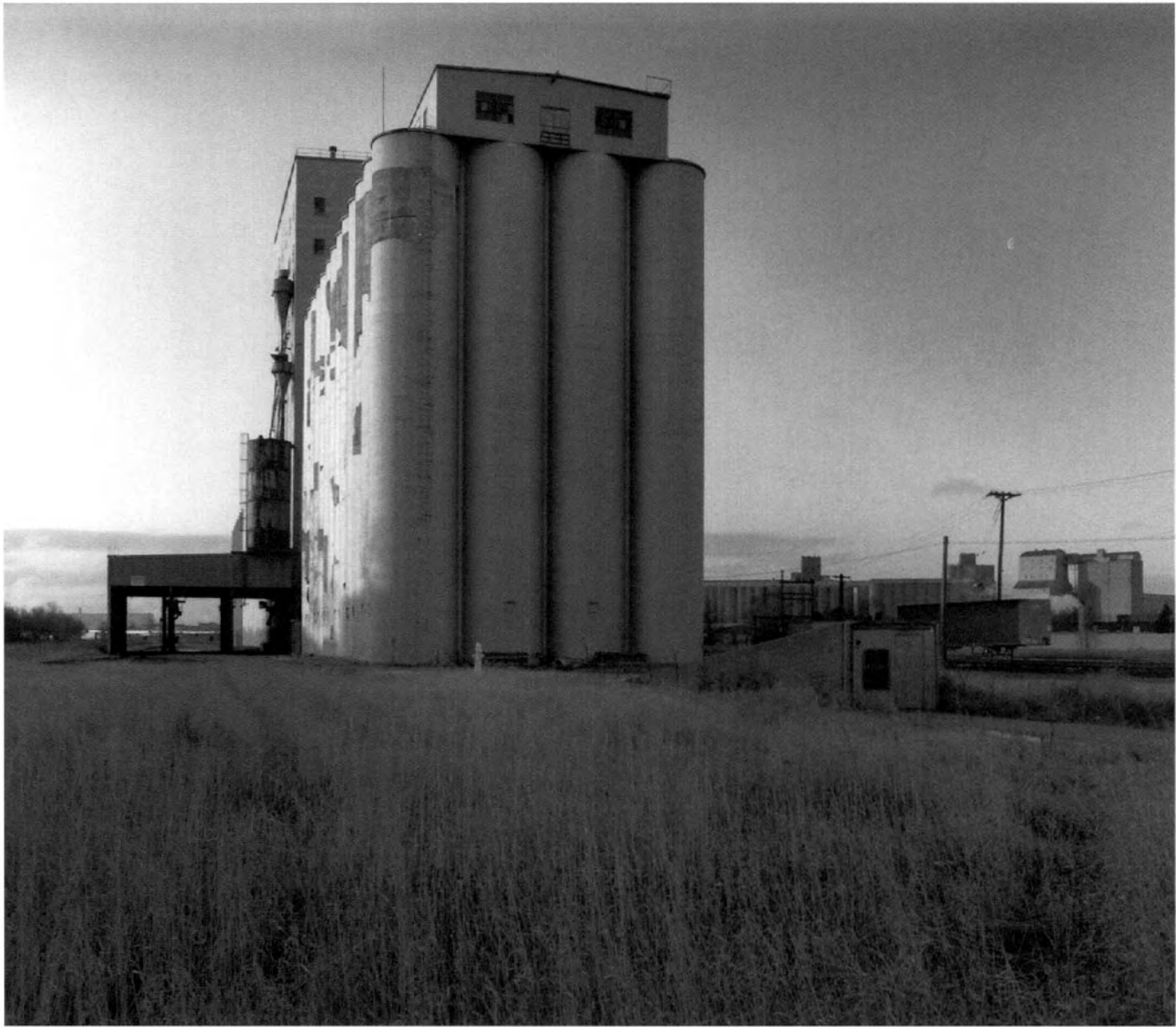
ABANDONED ELEVATOR, KASOTA AVENUE SOUTHEAST, MINNEAPOLIS, 1991
